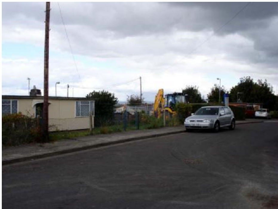
Fig. 3. Land at Old Barrow Hill, Shirehampton. The excavator is at the location of trench 2.
