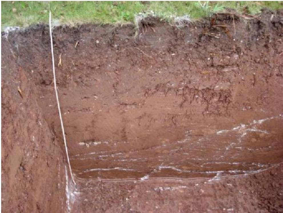
Fig. 6. Trench 3, showing calcite formations within the Triassic mudstones overlain by slope deposits consisting of gravelly clay.
